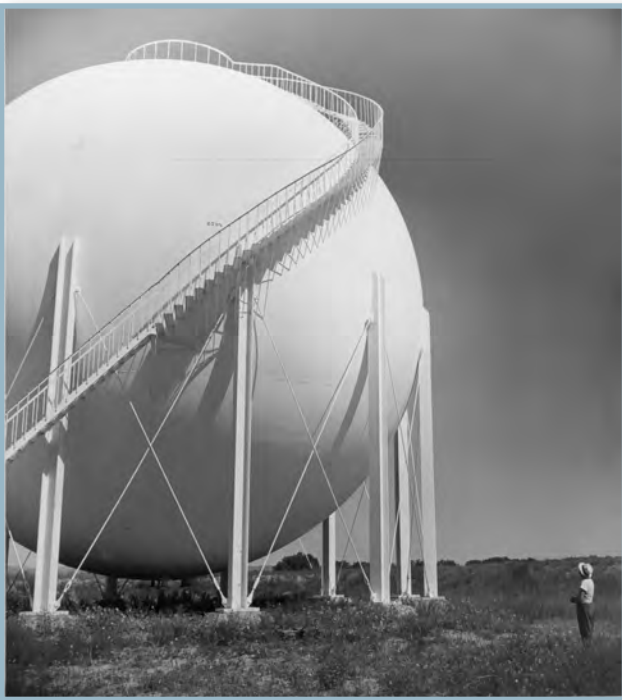
Natural Gas Storage, Somewhere in the Midwest, by Louise Putman Missouri State Archives, Louise and Omar Putman Photograph Collection
